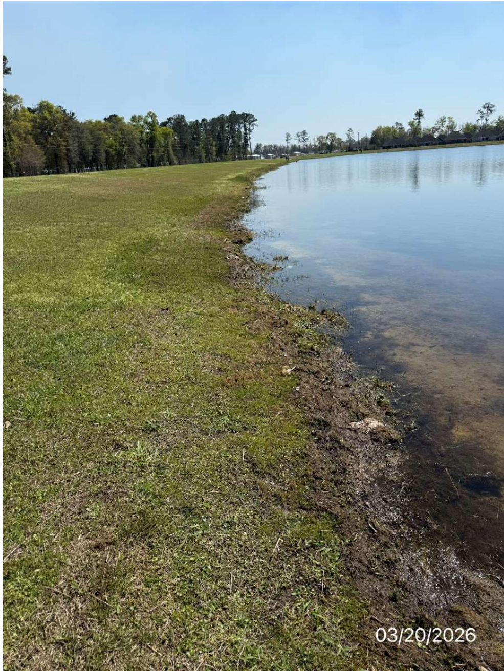
Picture #4 - Typical upstream slope condition.
