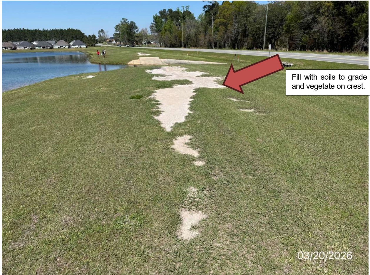
Picture #2 - Crest Condition south of the concrete spillway. Add soil and grass ( \pm 80' x 15')
