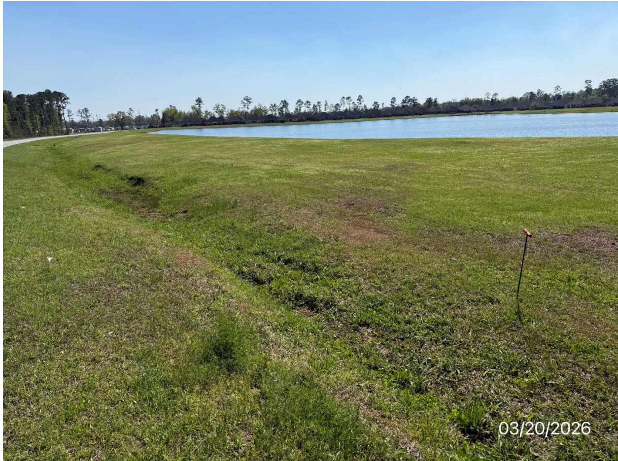
Picture #8 - Typical downstream slope.
