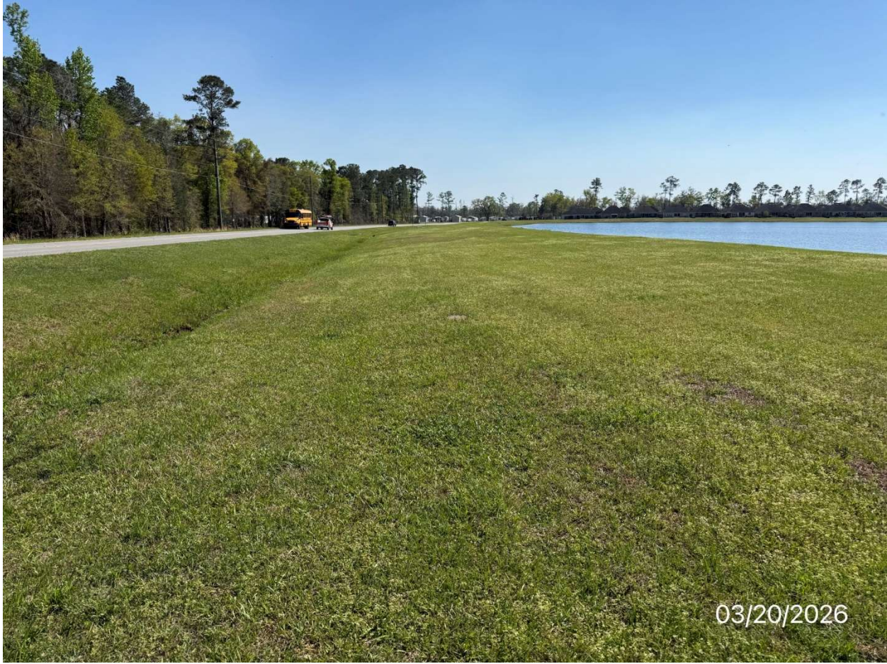
Picture #1 – Typical crest and backslope
