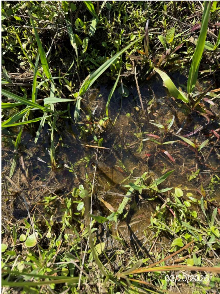
Picture #9 - Typical standing water in the ditch on the downstream slope at toe of the dam. Mostly hydrophilic vegetation on the ditch and the ditch does not drain well. Water is clear and is not flowing. See the attached location map.
